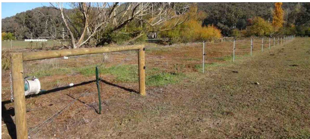
Figure 7.11 – Full-length sacrificial fence
