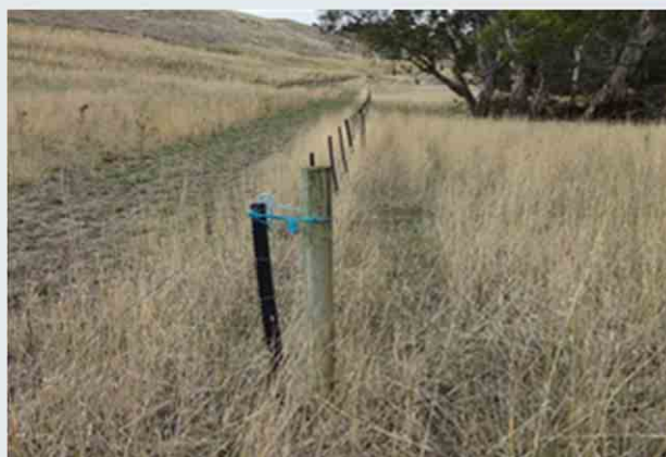
Figure 7.10 – Plastic droppers with metal insert for strength, connected to pine post by bale twine
