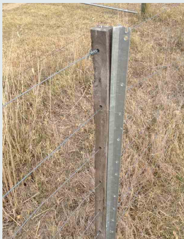
Figure 7.8 – A wooden dropper attached to a star picket
